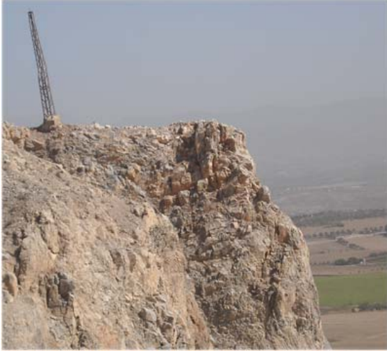
Figure 3: Overturned strata in the southern side of the rim of the Tigradou crater
